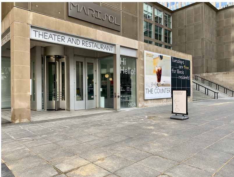
Accessible Entrance to the MCA Edlis Neeson Theater at the corner of Pearson and Meis Van Der Rohe Way. The entrance on the ground-level plaza has an automatic door, a revolving door, and a push-door exit.
